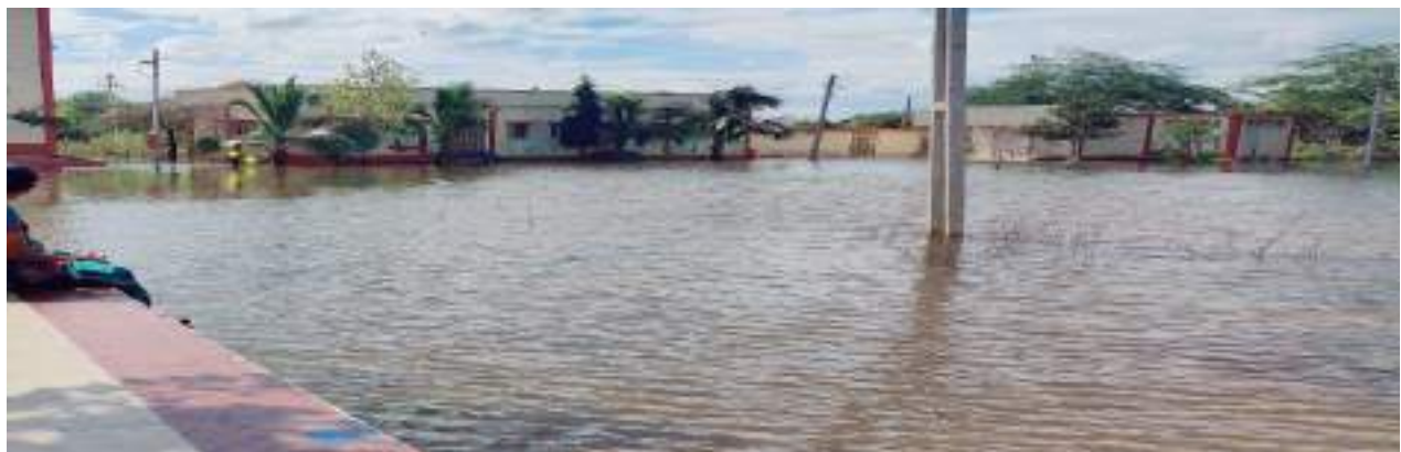
Water Storage due to rain water flow in the North West corner of the college campus
