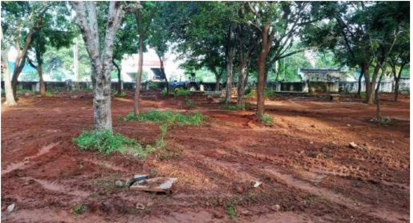
Landscape work in progress
